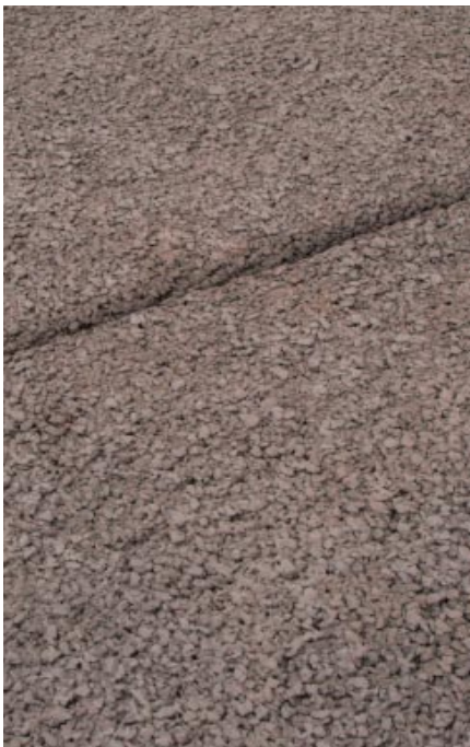
Above: Pervious Concrete (detail)
