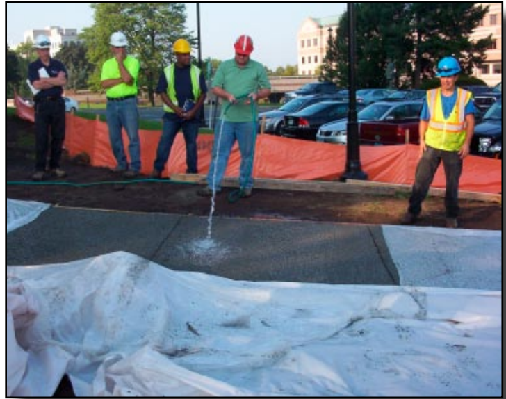
Above: Testing Porosity of Pervious One Day After Placement
