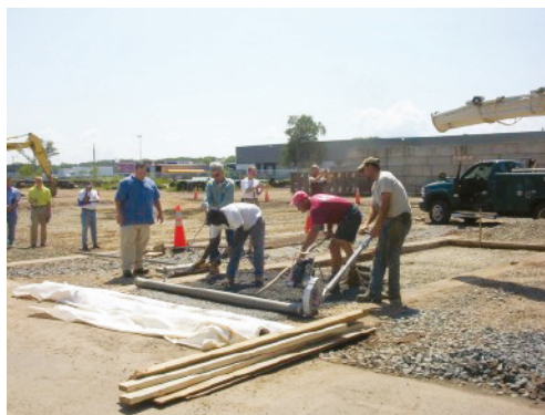
Pervious Concrete Placement at MDC's Maxim Road Facility
