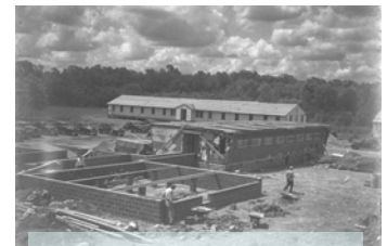
UCONN Dorms 1947 Under-Construction
