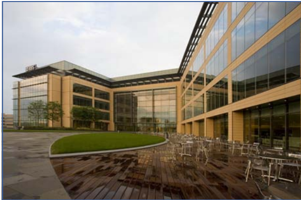
New Large Construction '10 RBS Americas H Q Turner Construction
