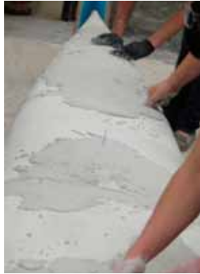
Figure 9: Applying First Layer of Concrete
