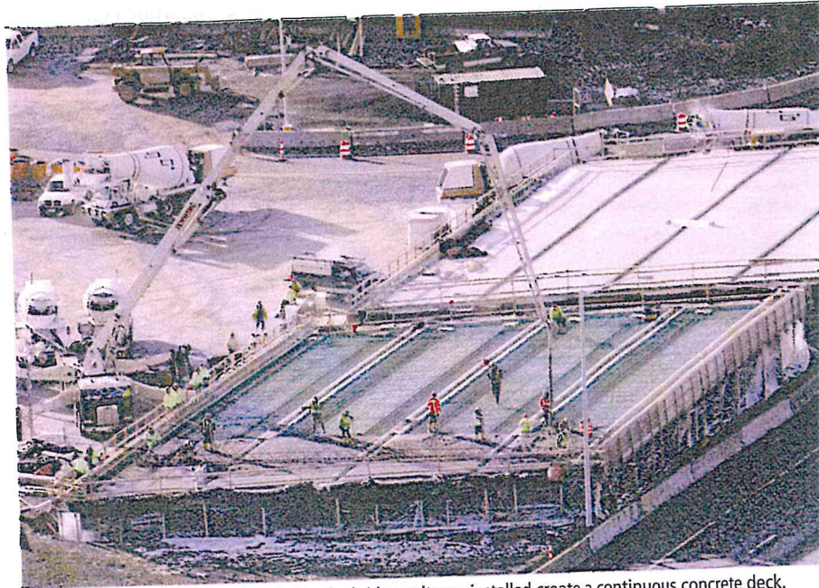
» Longitudinal closure pours placed after the bridge units are installed create a continuous concrete deck.
