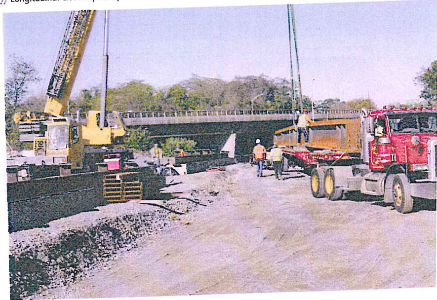
» Longitudinal closure pours placed after the bridge units are installed create a continuous concrete deck.
