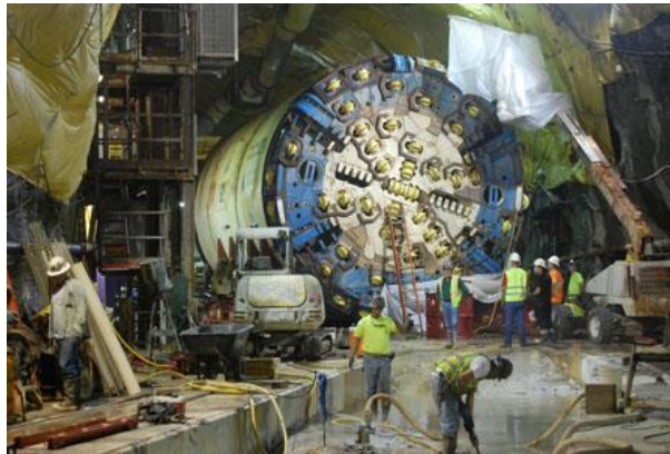
TBM in chamber - production to 391'/week;
